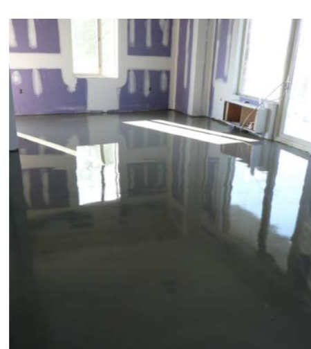
A high output means even large-area screed surfaces are no problem for the SLU PRO 80.
