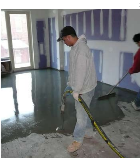
When processing self-leveling underlayment, the SLU PRO 80 shows its strengths – the surface becomes horizontal and flat with almost no other intervention.
