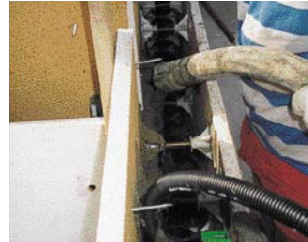
In addition to standard operations such as base-coat plastering or spray plastering, the P 13 is excellently suited for use where large volumes must be pumped, for example, when infilling formwork.
