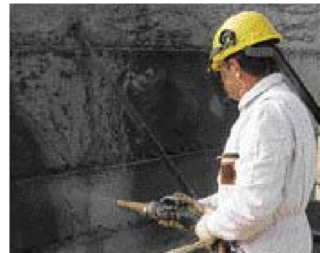
Coarse-grain shotcrete (here 8 mm) can only be handled using a P 13 type piston pump.
